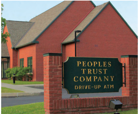
Enosburg Falls 140 Main Street Enosburg Falls, VT
